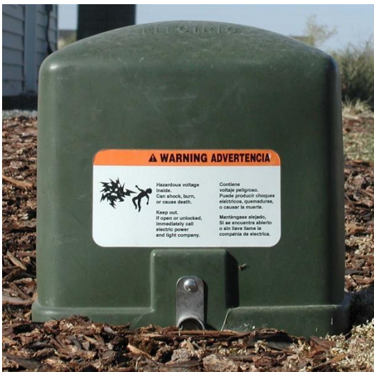
Figure 2. Secondary Above Ground Pedestal (MO-PED) and Transformer
