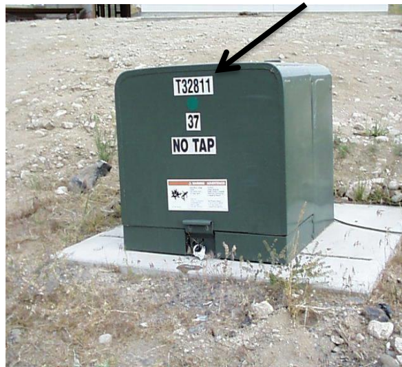
Figure 2. Secondary Above Ground Pedestal (MO-PED) and Transformer
