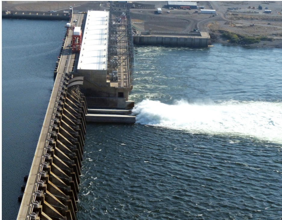
Figure 2 Priest Rapids Fish Bypass in operation, April 2014.
