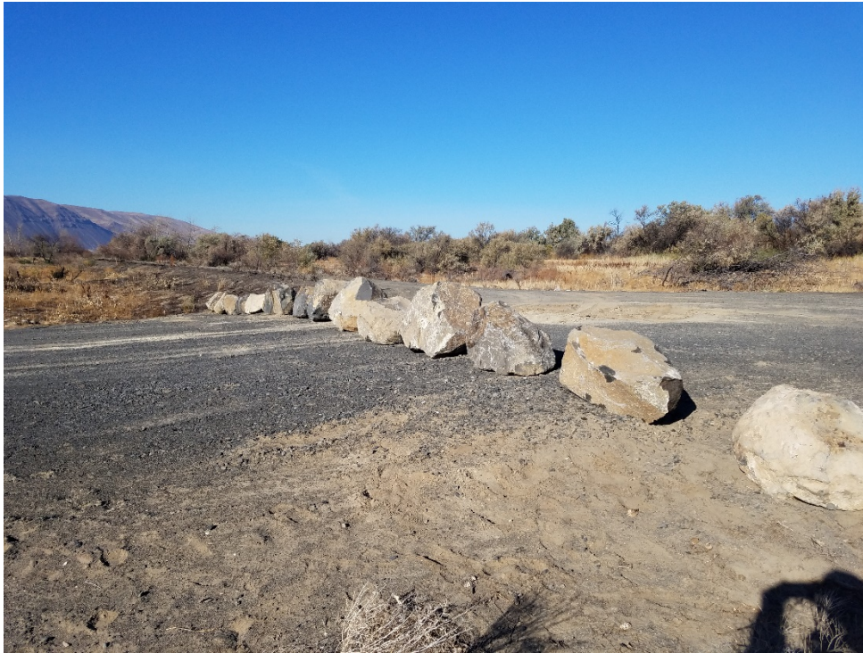
Figure 4 Example of boulder barrier placed along Crab Creek.
