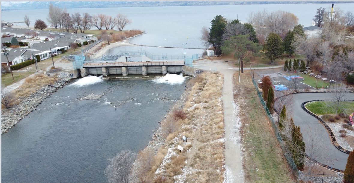
Figure 2: Okanagan Lake Outlet Dam.
