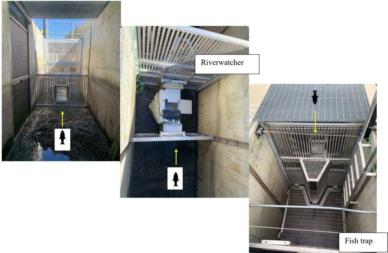
Figure 5: Fish trap (with Riverwatcher) example from the Samish River, WA.
