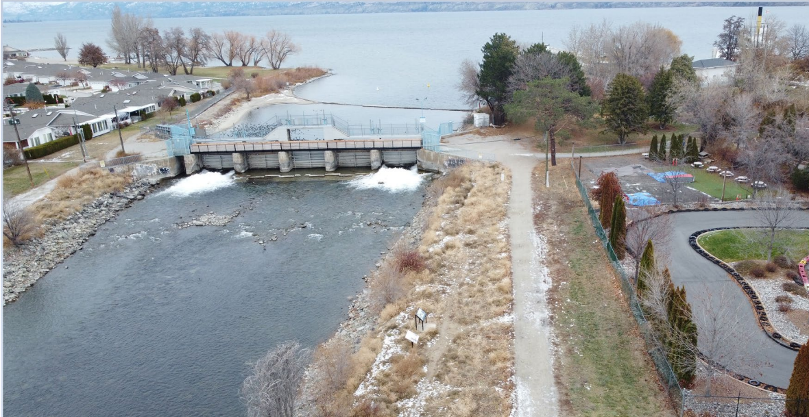
Figure 2: Okanagan Lake Outlet Dam.
