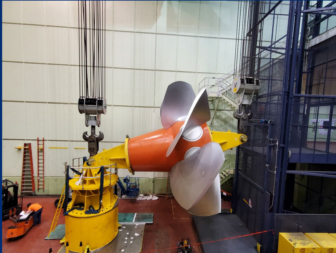
PR Unit Rehab (P1), Turbine Flip.
