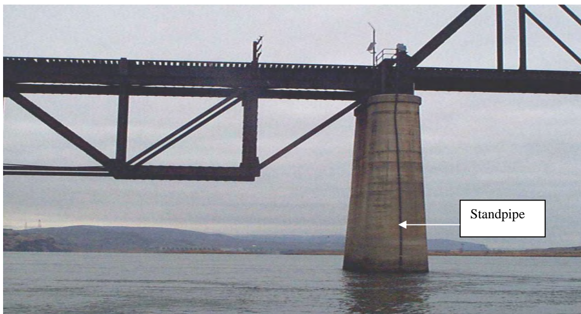
Figure 7 Photograph of Wanapum dam tailrace water quality fixed site monitoring station, looking upstream at Beverly Bridge. Priest Rapids Project, mid-Columbia River.
