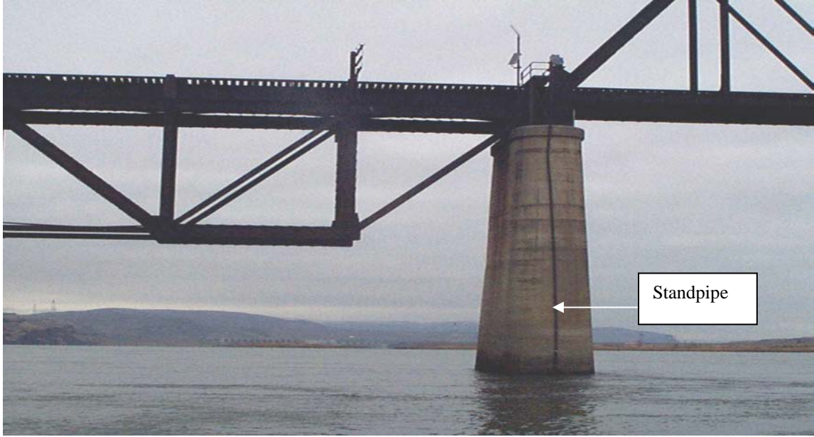
Figure 7 Photograph of Wanapum Dam tailrace water quality fixed-site monitoring station (FSM station), looking upstream at Beverly Bridge. Priest Rapids Project, mid-Columbia River.
