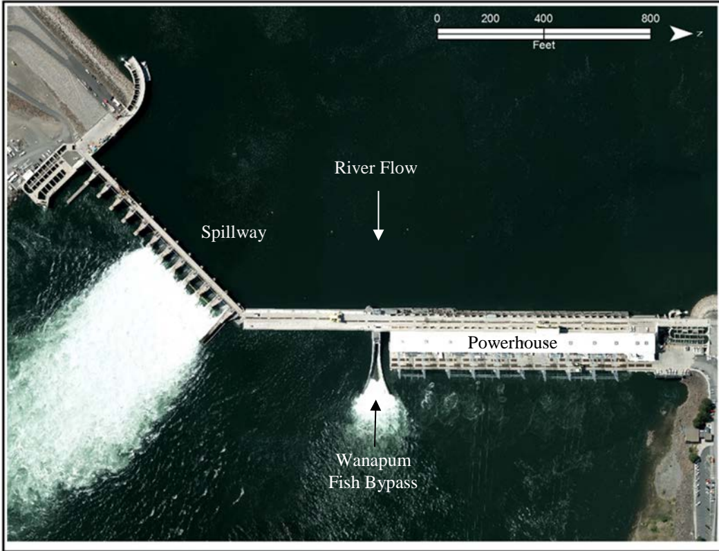
Figure 2 Aerial photograph of Wanapum Dam, mid-Columbia River, WA.
