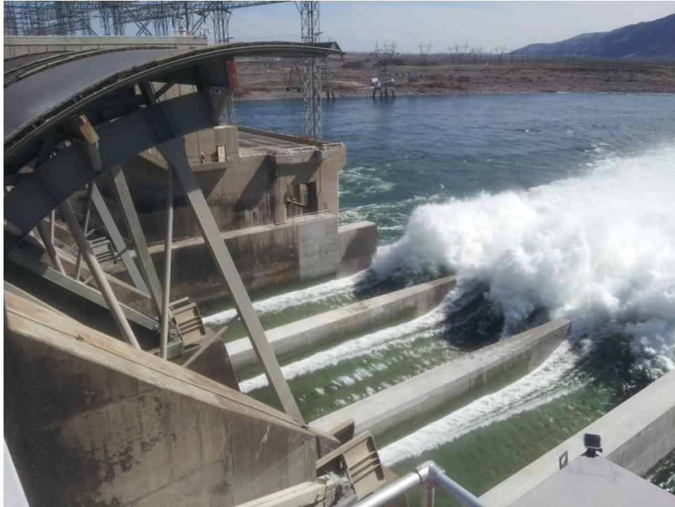
Figure 6 Priest Rapids Fish Bypass facility, mid-Columbia River, WA.
