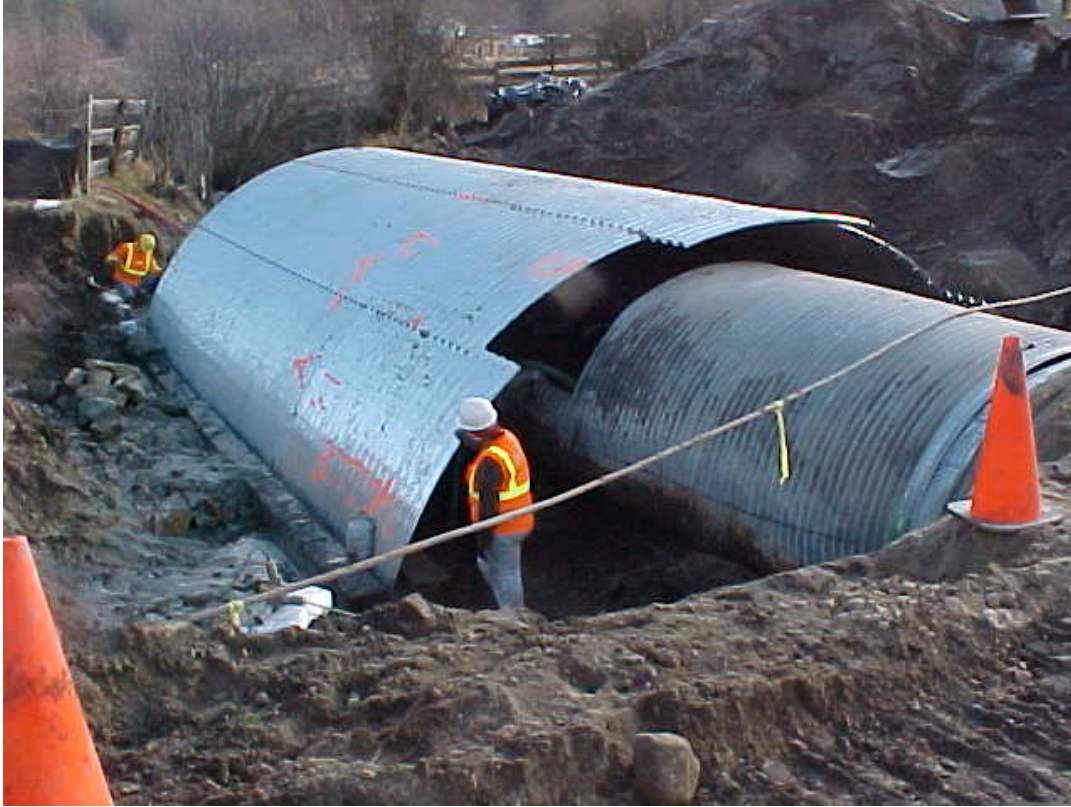
Figure 4 Culvert at RM 15 during installation.
