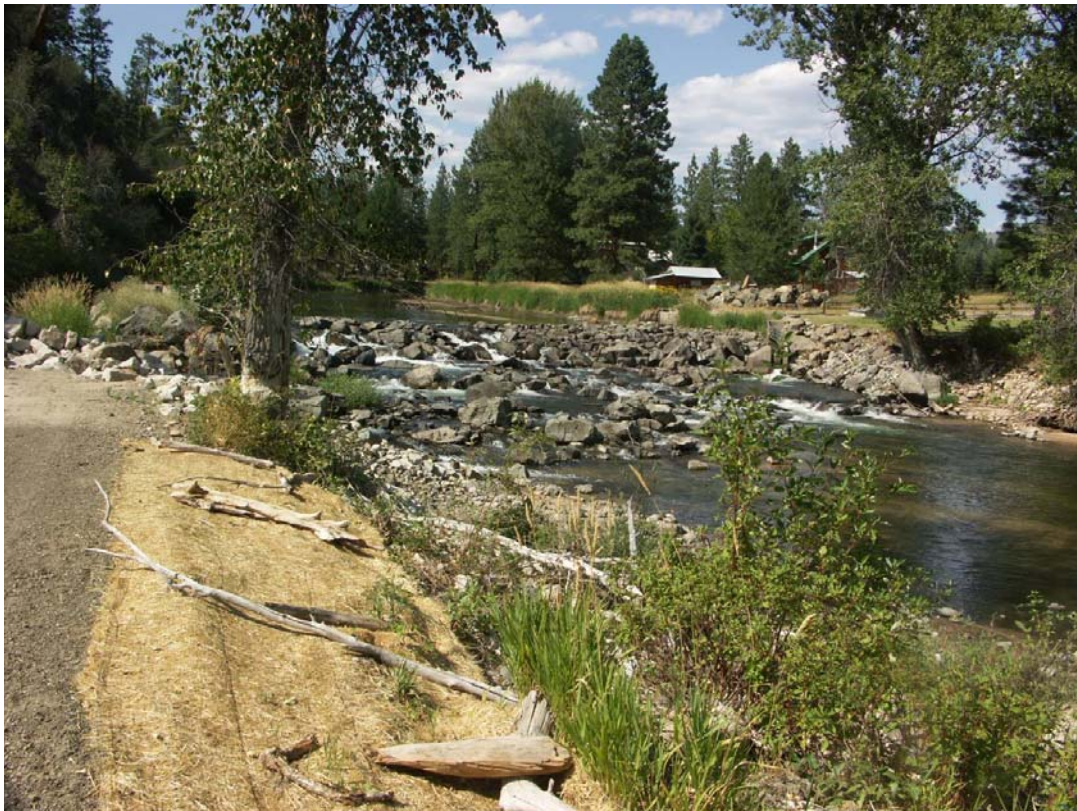
Figure 1 The Fulton diversion dam site prior to construction.
