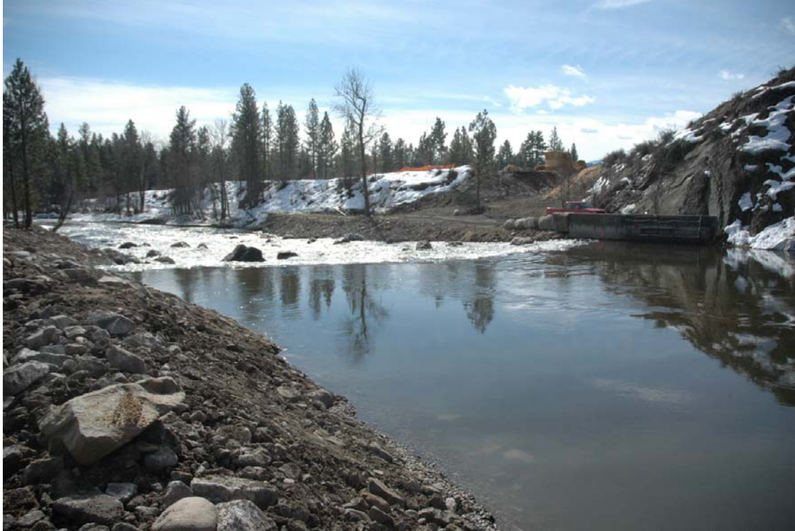
Figure 2 The Fulton diversion dam site after construction in April 2007.
