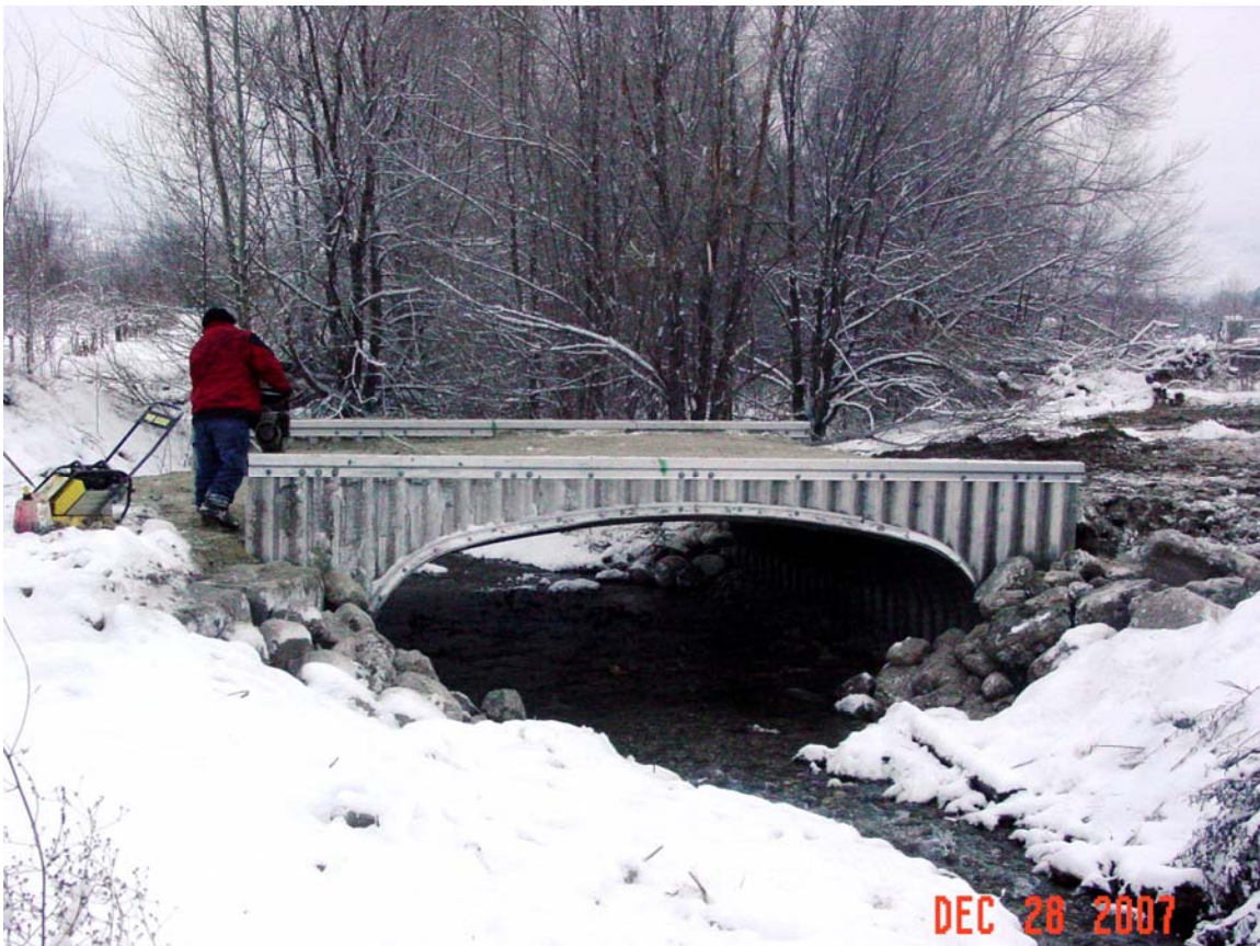
Figure 12 Antoine Creek culvert upon replacement.
