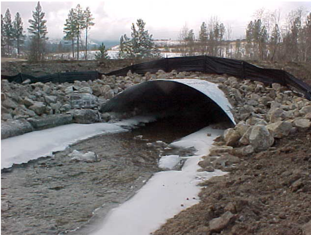
Figure 5 Culvert at RM 15 after installation.
