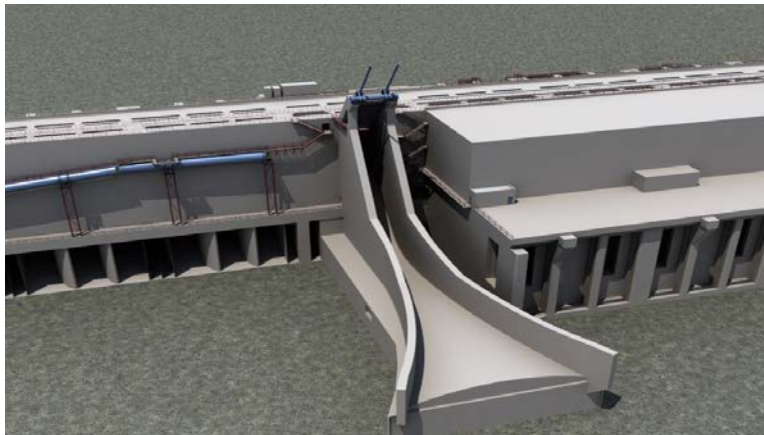
Figure 1. Graphic diagram of the Wanapum Fish Bypass (WFB) showing the downstream exit.
