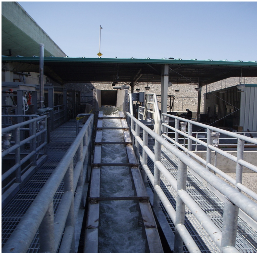
Figure 8 Steppass fishway section of the off ladder adult fish trap located at Priest Rapids Dam, Columbia River mile 397-1, Washington, USA.
