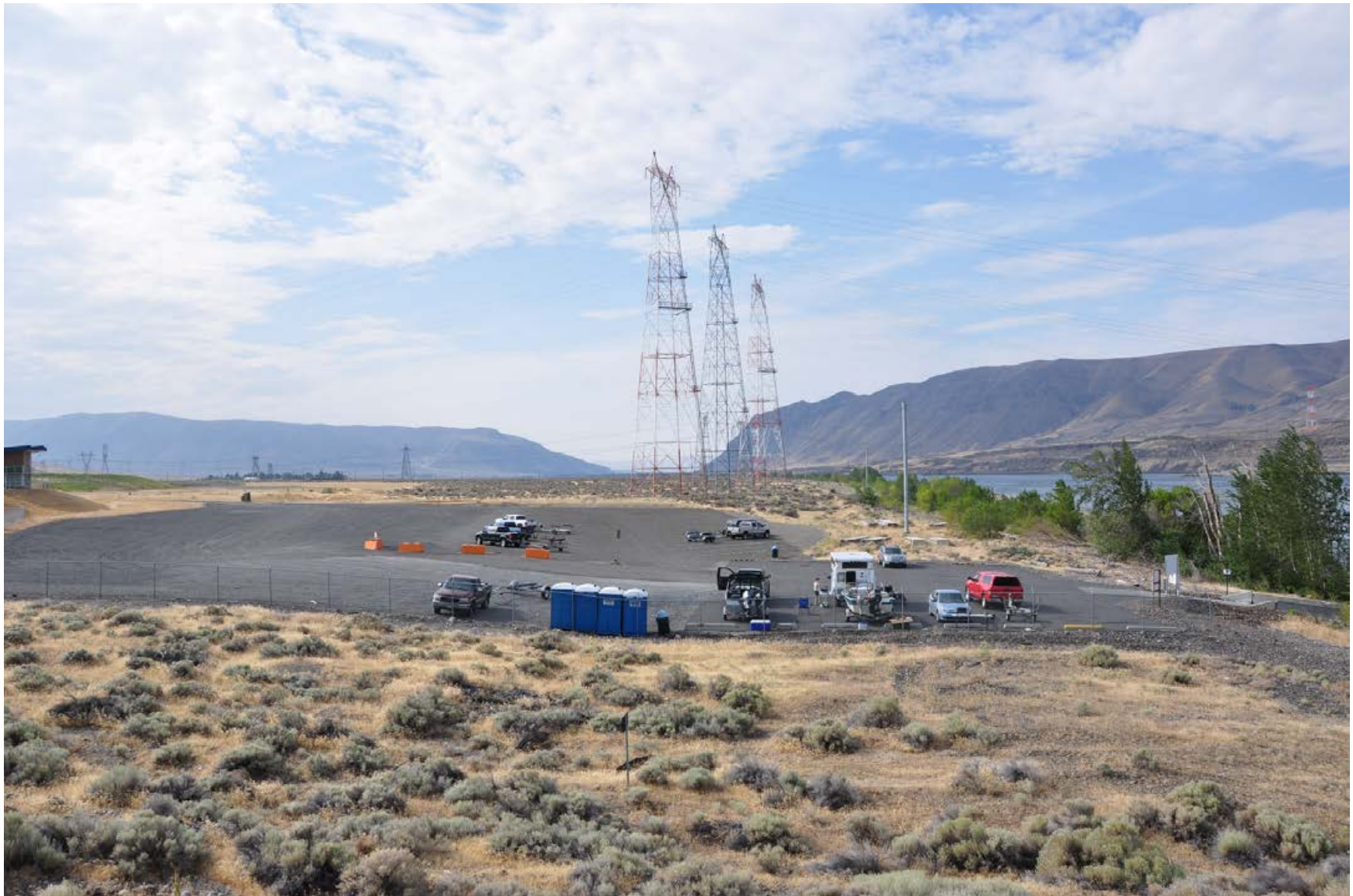
Wanapum Dam Lower Boat Launch
