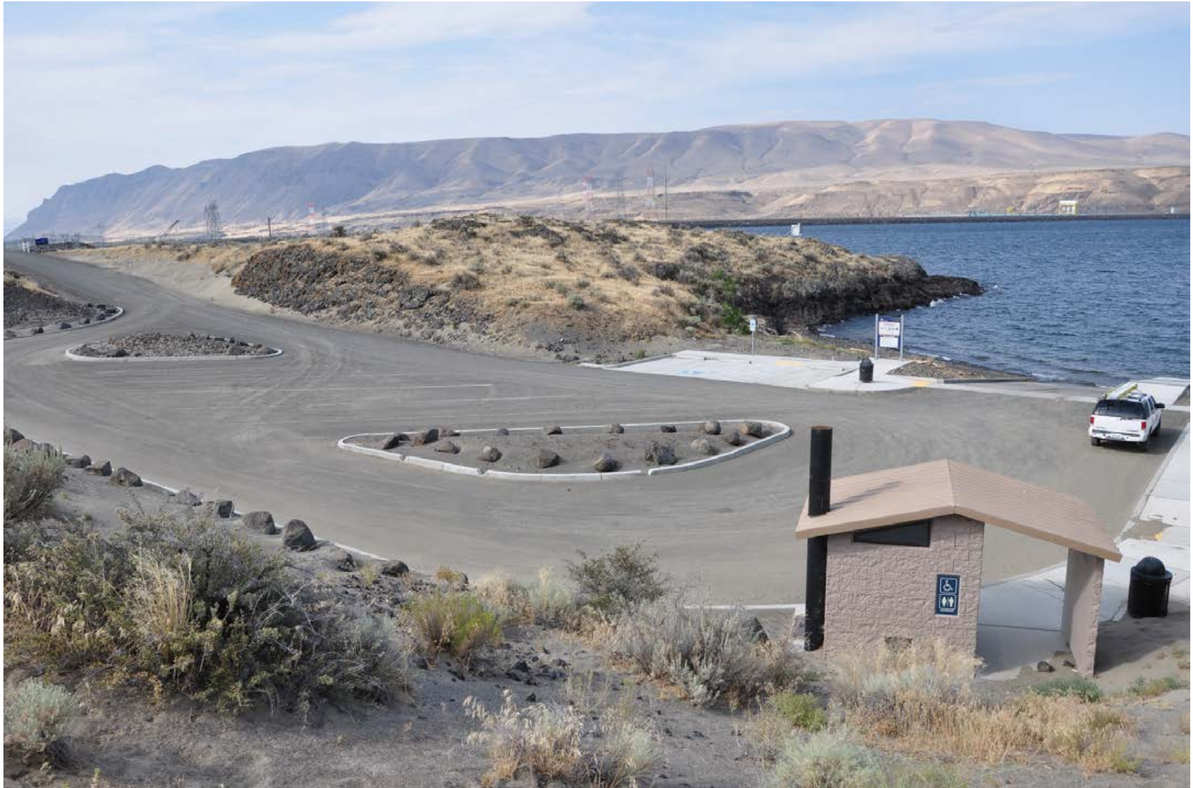
Wanapum Dam Upper Boat Launch
