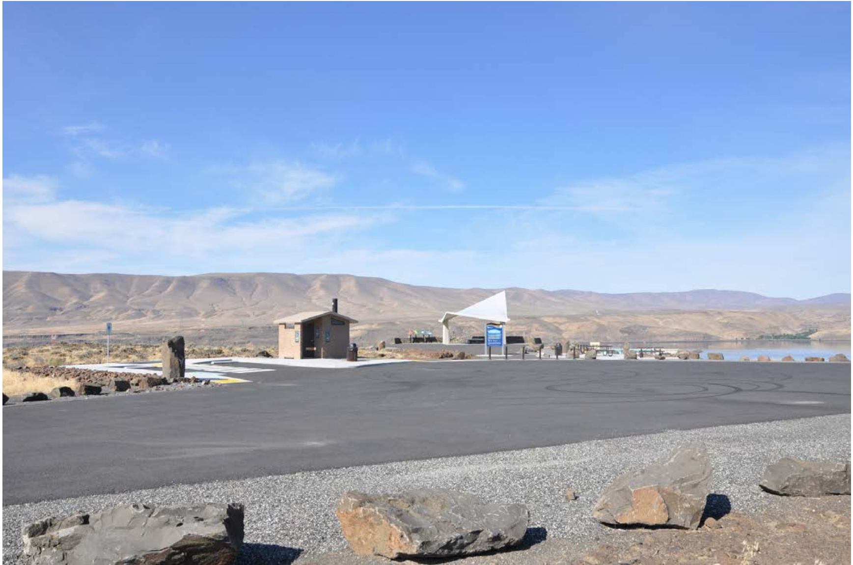
Wanapum Dam Overlook
