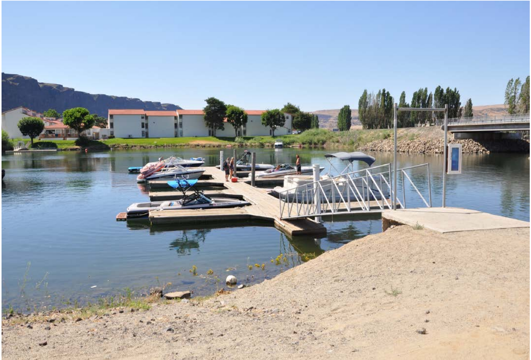
Crescent Bar Marina
