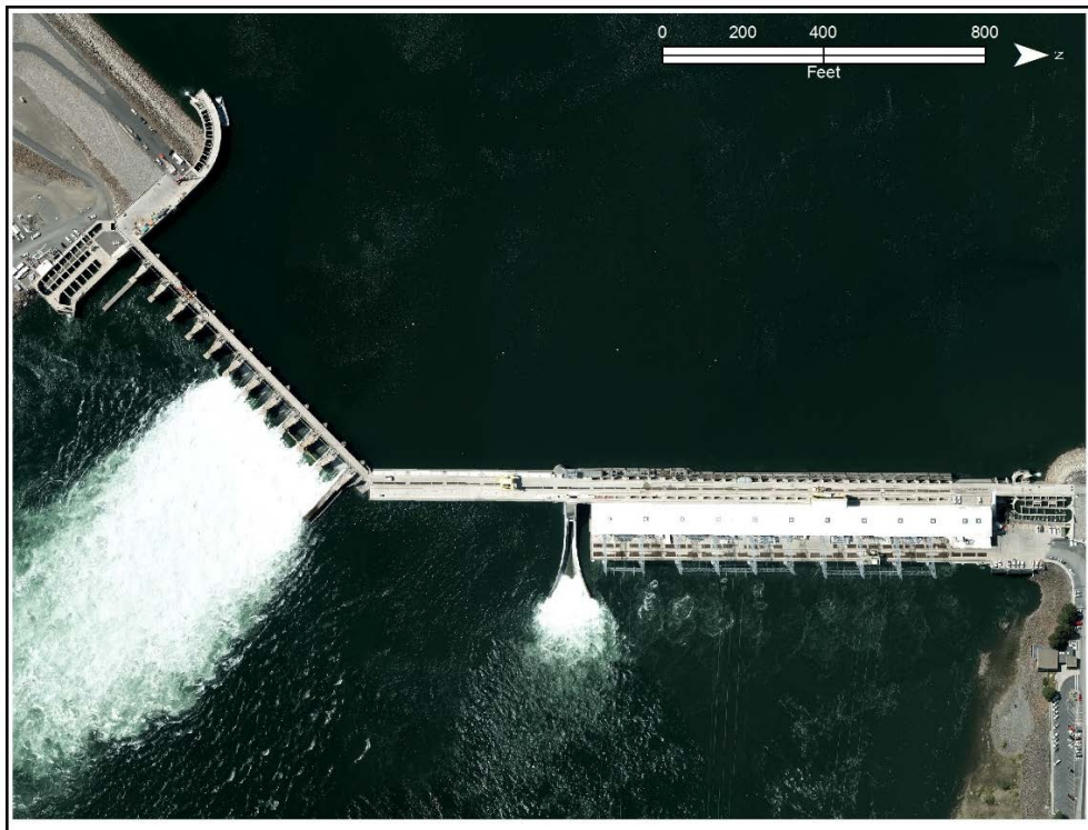
Figure 3 Aerial photograph of Wanapum Dam, Priest Rapids Hydroelectric Project, mid-Columbia River, WA.
