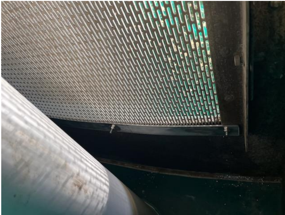
Figure 3. Sump screen fix viewed from the outside of a circular tank.
