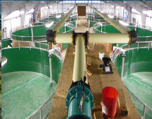
Carlton Acclimation Facility
